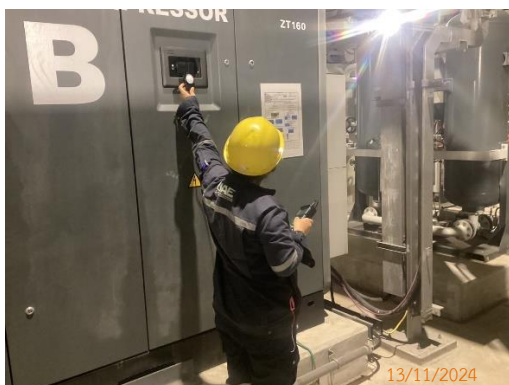
INSTRUMENT AIR COMPRESSOR
